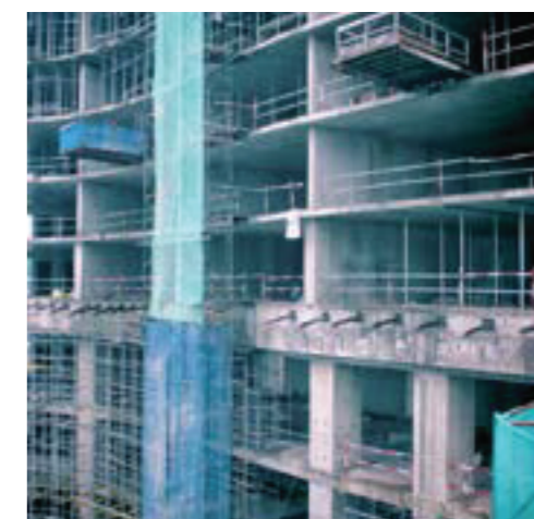
Transfer slab of Hilton Danang - 2015
